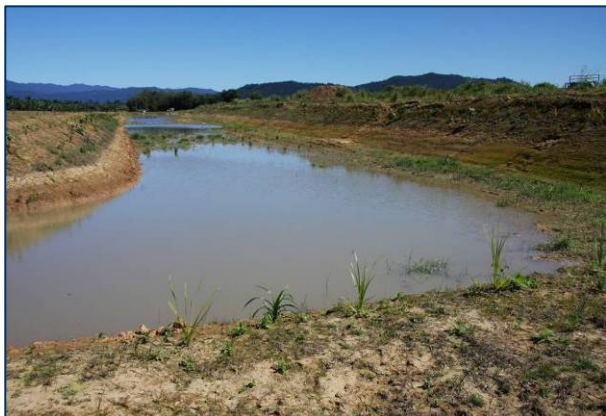
The 2.45 hectare wetland designed and built to treat run-off from the banana farm. Photo: DEEDI
